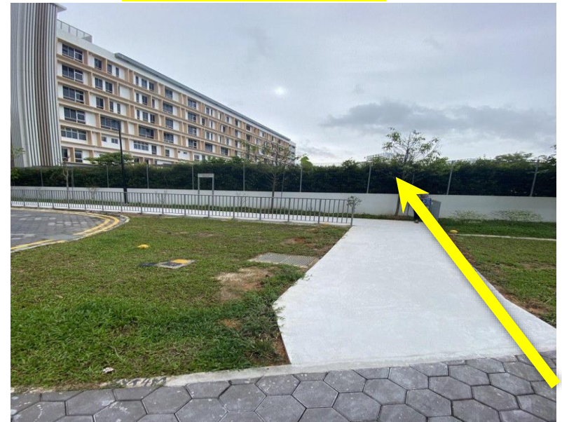
Access to footpath from Block 627B leading to Gate 2
